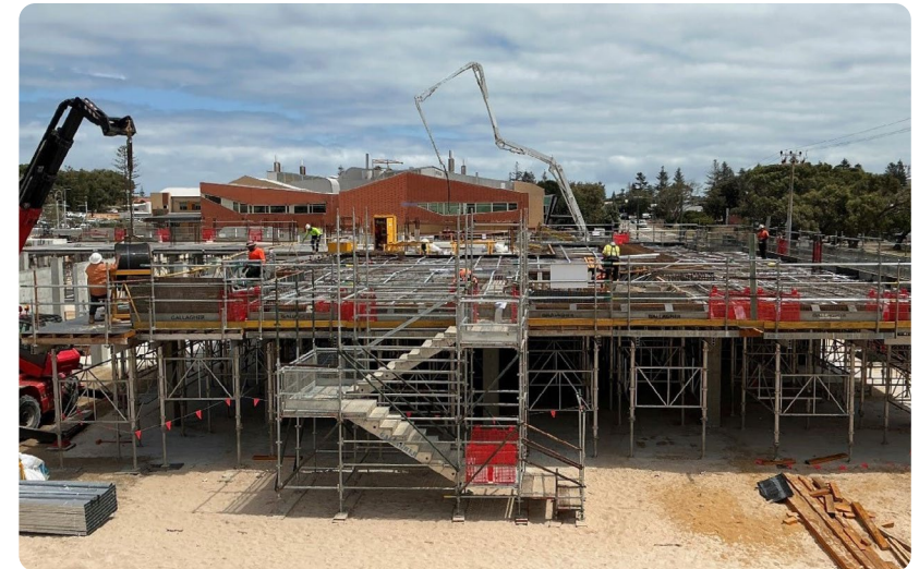
● Geraldton Health Campus redevelopment, October 2024.
