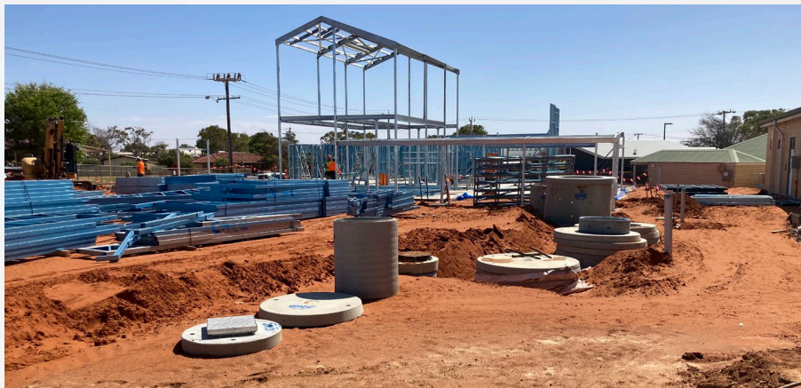
Picture 1. Wall trusses and plumbing works installed on site
